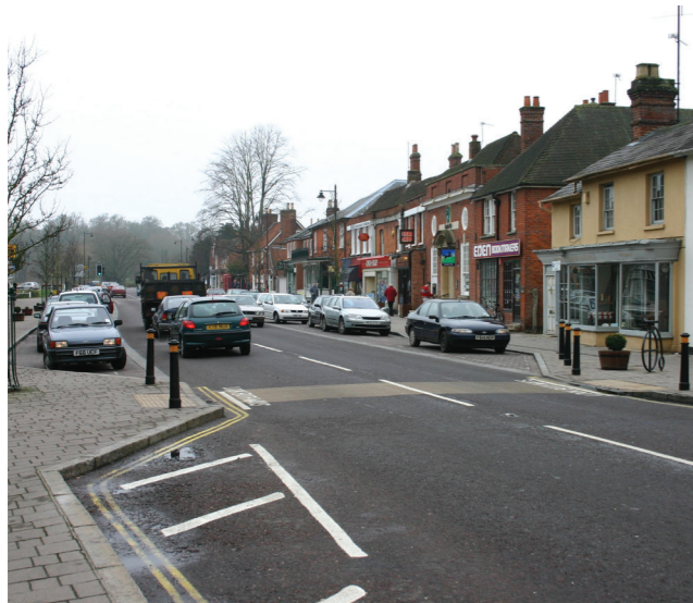
Carriageway narrowing at an informal crossing
